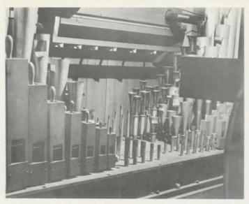
Solo Chamber: Front to back: Tibia, Tuba Mirabilis, Brass Sax. Bass drum in lower right corner.
